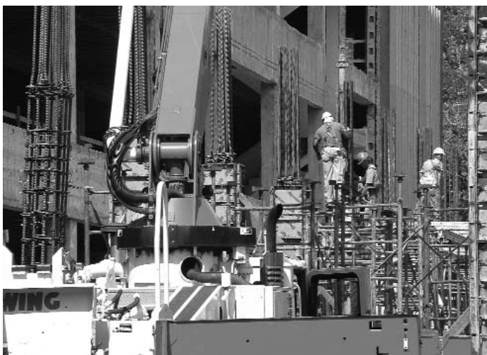
Simultaneous concrete work and demolition have been in progress for the past several months at Library West
